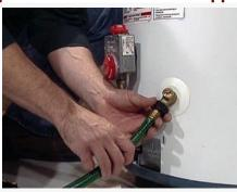
If you have an electric water heater, turn off the power at the breaker-box. If yours is a gas heater, turn the thermostat to the "pilot" setting. Connect a hose to the drain valve located close to the thermostat, but don't open the valve yet. Turn off the coldwater supply that feeds the water-heater.
