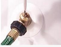
Inside your house, open up one of the hotwater faucets in one of your sinks or tubs. This will prevent a vacuum from forming in the lines. Go back to the water-heater, and open the drain valve to drain the hot water out of the tank. Make sure the far end of the hose is draining somewhere that won't be harmed by hot water. An outside driveway is ideal.
